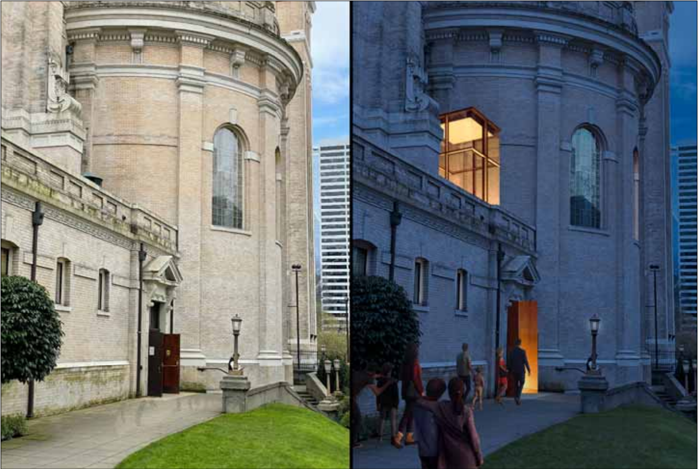
Left: the entry as it currently appears. Right: a rendering of the entry as it will appear in early evening, with the “light monitor” above the entrance and the doors standing open. One goal of the project is to make it clear to visitors that this is a substantial entry point for the Cathedral.
